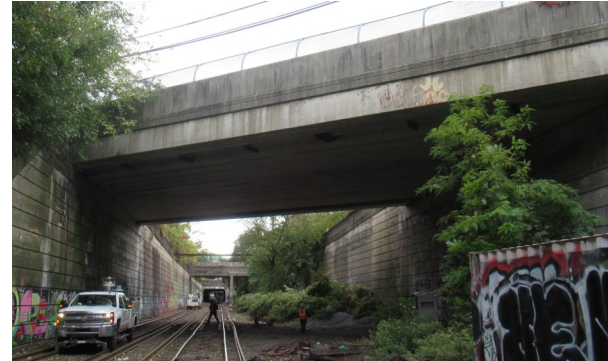
CSX tracks below 69 th Street Bridge
