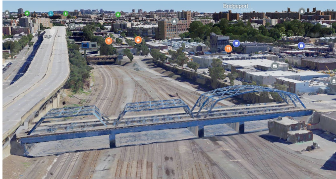
CSX tracks below Leggett Avenue Bridge
