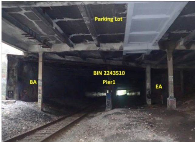
Flatbush Ave. Bridge
