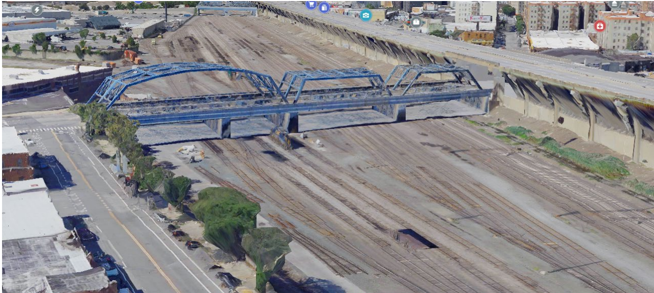
Amtrak tracks below Leggett Avenue Bridge
