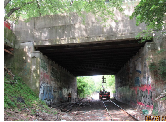
McDonald Ave. Bridge
