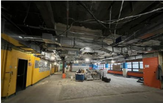
1-General condition on ground floor with exposed historic finishes and exposed steel and new ductwork
