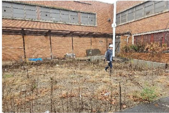
2-Building entrance canopy
